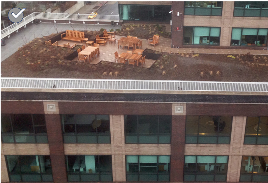
A rooftop terrace could offer an amenity to residents or employees.
