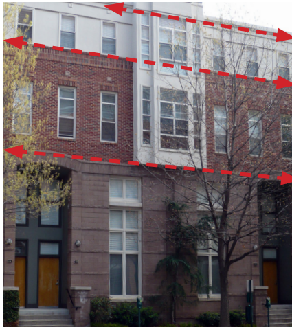
Express the floors of a building in a way that is compatible with the floor expression of other traditional buildings on the block.
