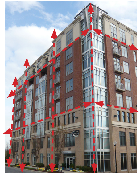
Articulate a building mass to include vertical and horizontal elements that relate to the proportions of nearby traditional buildings.
