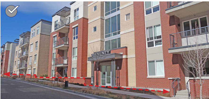
Step the first floor of a building along a sloped street to maintain a constant street presence.
