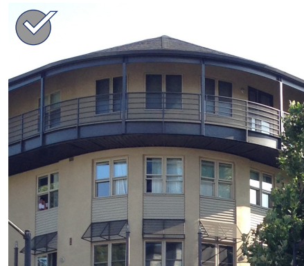
Design a roof to be architecturally consistent with the overall architectural design and detailing of the structure.
