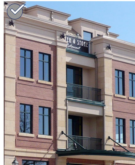
Design a window to create depth and shadow on a façade. This is particularly relevant in the Downtown Core and Tuning Fork Character Areas.
