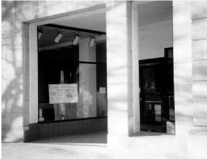
Illustration M - Commercial Architectural Detailing. Doors and door openings protected by architectural recesses.
