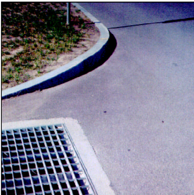
Curb-cuts should not be used for driveways in the Elmira Road - Meadow Street Corridor.
