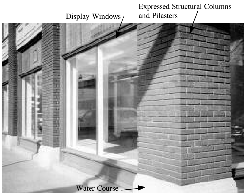
Illustration N - Commercial Architectural Detailing. Characteristic local commercial architectural detailing, including primarily masonry materials.
