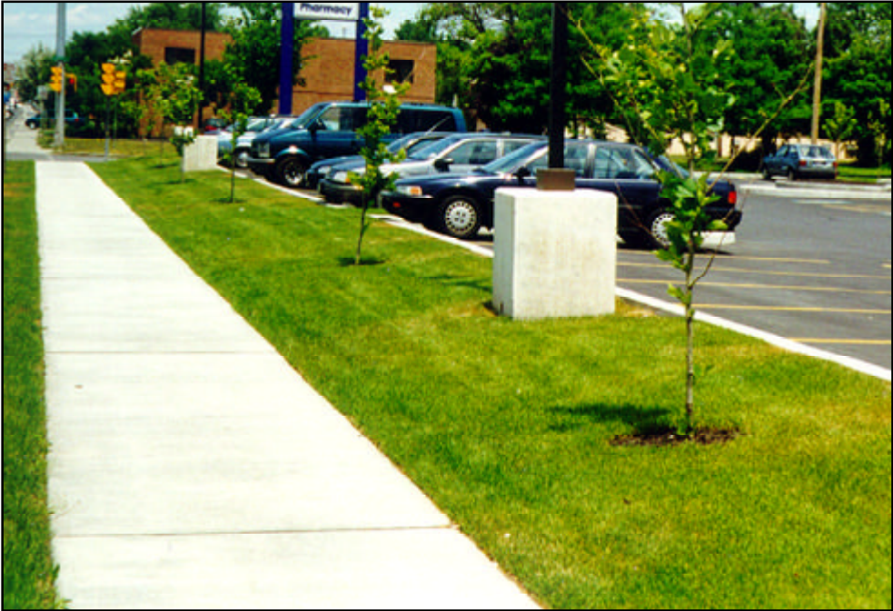
Illustration DD - An example of 5'-0" concrete walk in the Meadow Street right-of-way.
