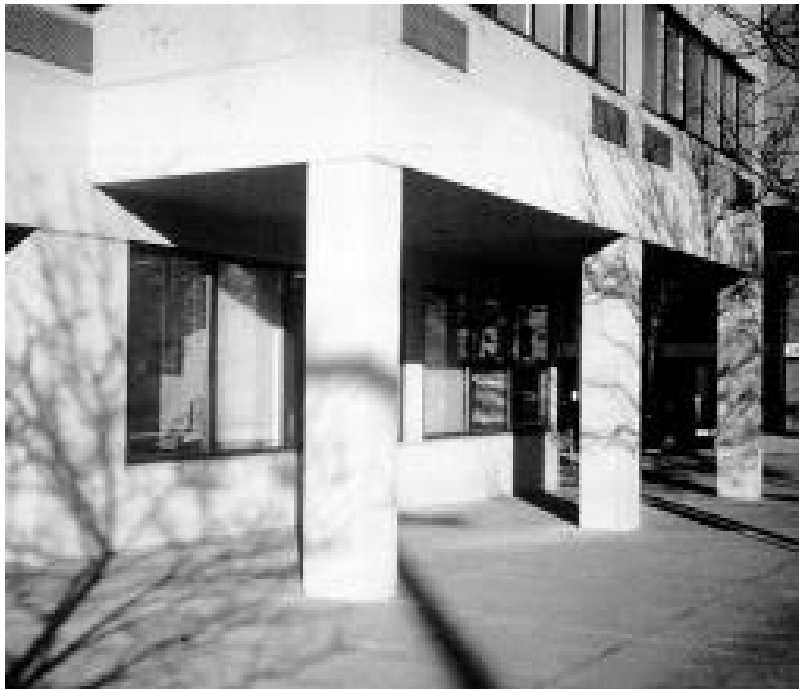
Illustration O - Commercial architectural detailing, to include arcades, providing building character as well as protecting pedestrians from wind and precipitation at entrances and display windows.
