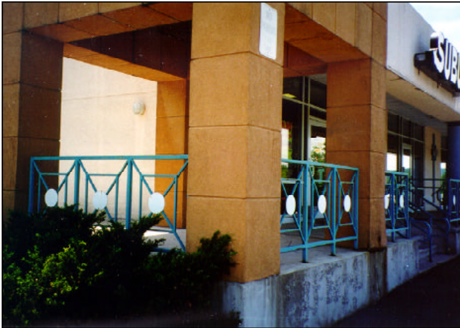
Illustration JJ - An example of a rehabilitated building, conforming to primary facade having not less than 35% of windows, awnings and arcades.
