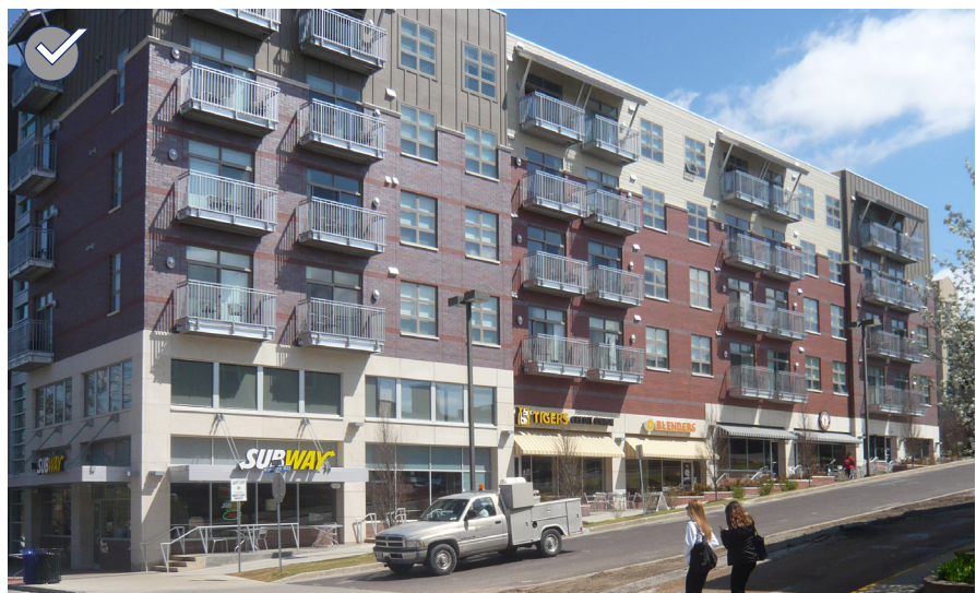
Step the first floor of a building along a sloped street to maintain a constant street presence.
