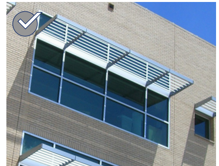
Consider including a building design feature that conserves energy, such as a window pergola/sun shading device.
