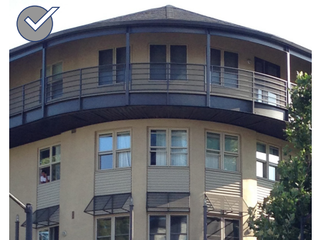
Design a roof to be architecturally consistent with the overall architectural design and detailing of the structure.
