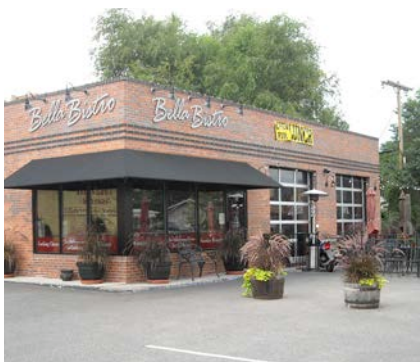
Seek opportunities for adaptive reuse in an existing building.
